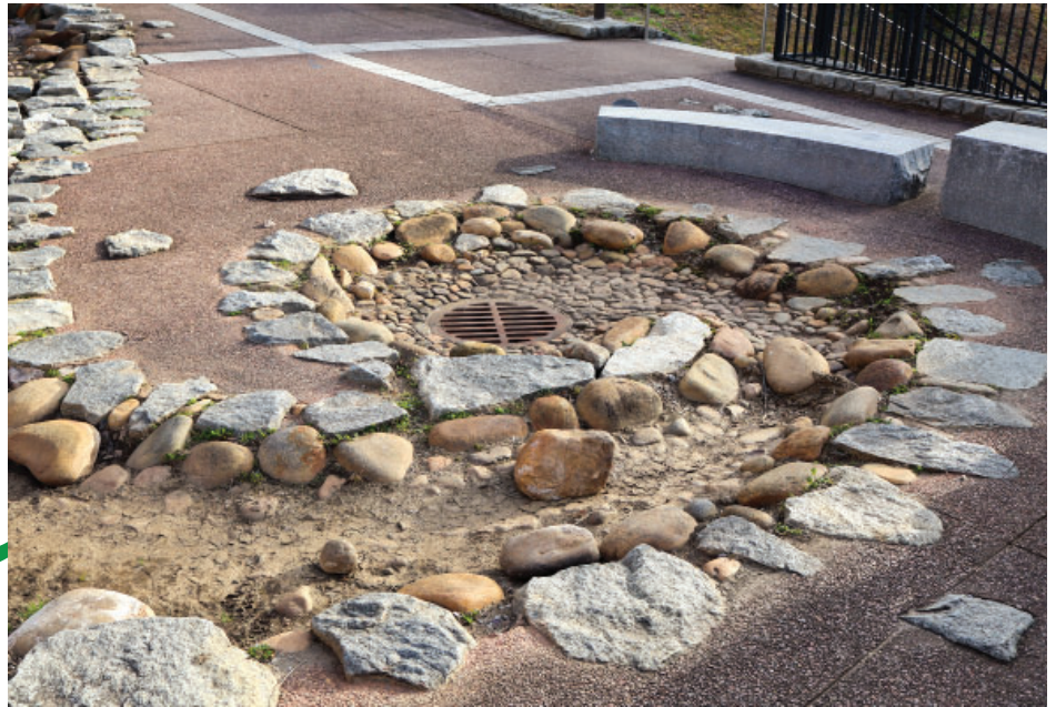
Decorative Drainage // Photo by Madeline Weller
